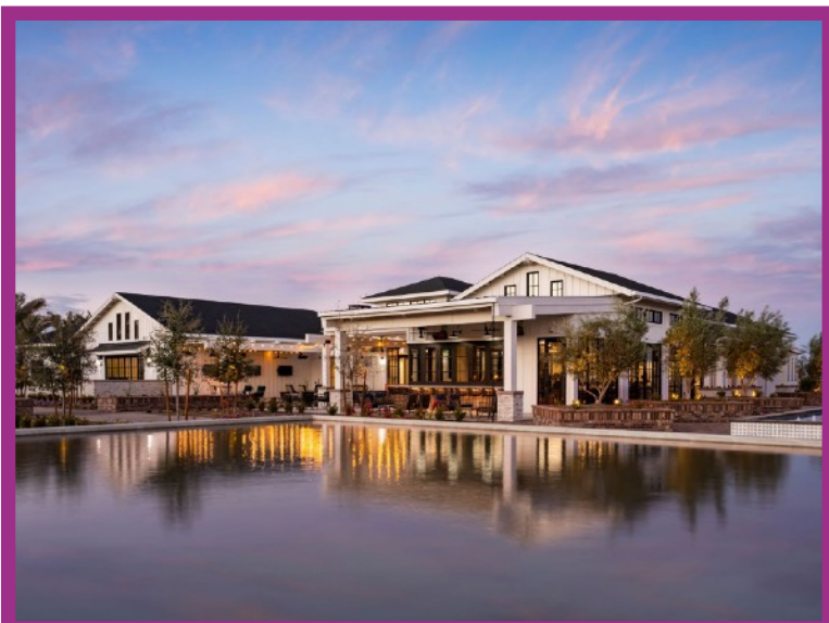
Sterling Grove By: Toll Brothers Signage: MSI Landscape Architect: Creative Environments
